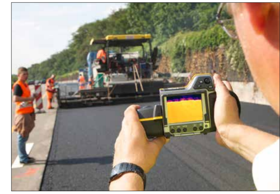
Even temperatures and optimal distribution of grain sizes result in a high quality asphalt surface.
