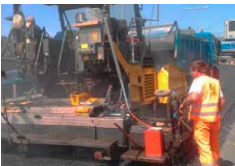
Autobahn A 100 in Berlin The most used road in Europe. Special features: Application of Porous Mastix Asphalt (PMA)
