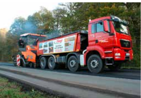
District administration Bielefeld Special features: Asphalting in avenues.
